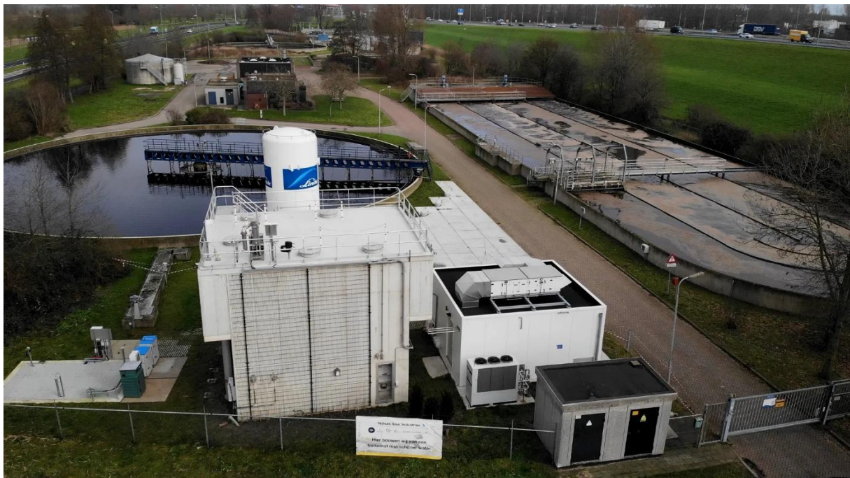
Figura 1 – View of the MicroOxi ozone treatment system at WWTP Houten.
